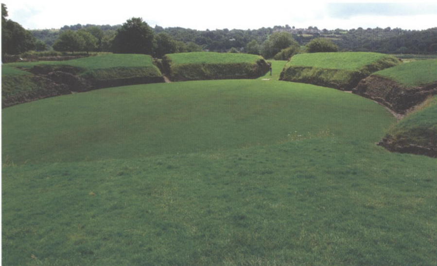
Roman amphitheatre in Caerleon. It is the only fully excavated amphitheatre in the United Kingdom, and an excellent example of a military amphitheatre. Built AD 90, it has a 56×41m arena dug into the ground. The encircling embankment was made from the dug-up earth and faced with stone. A 9-high timber superstructure crowned the embankment and held seating. The amphitheatre housed about 6,000 spectators, which little outnumbered a legion. It was not only used for gladiatorial games and venatio but also for legionaries' parades and training. (Author's collection)
